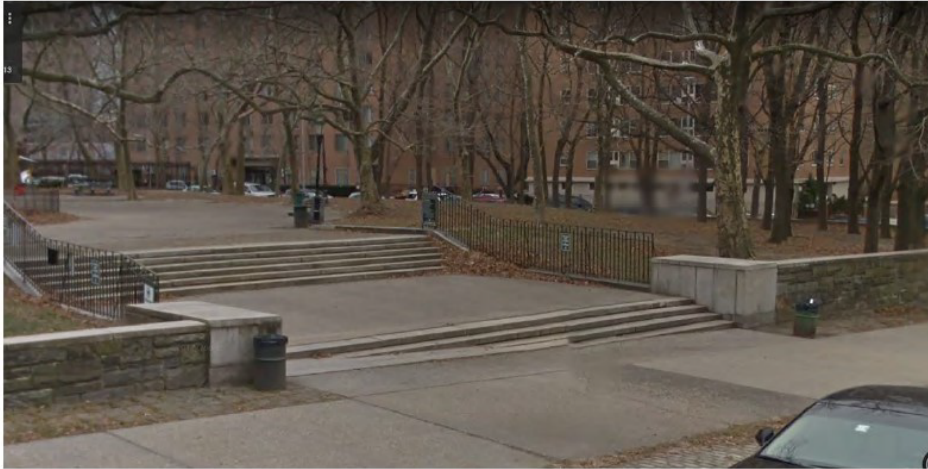
Myrtle Avenue Entrance Area - Existing Condition
