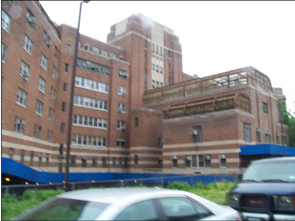
Photo 1: Building G (project site) from the Southwest
