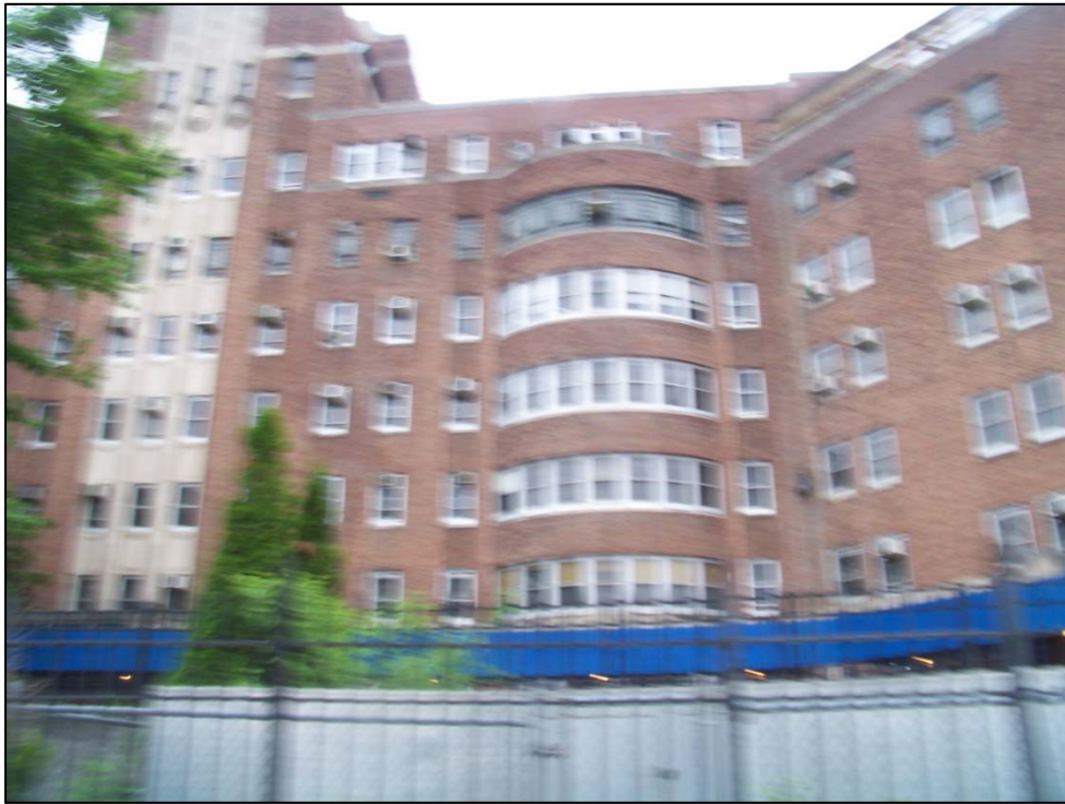
Photo 3: Building G (project site) from the North
