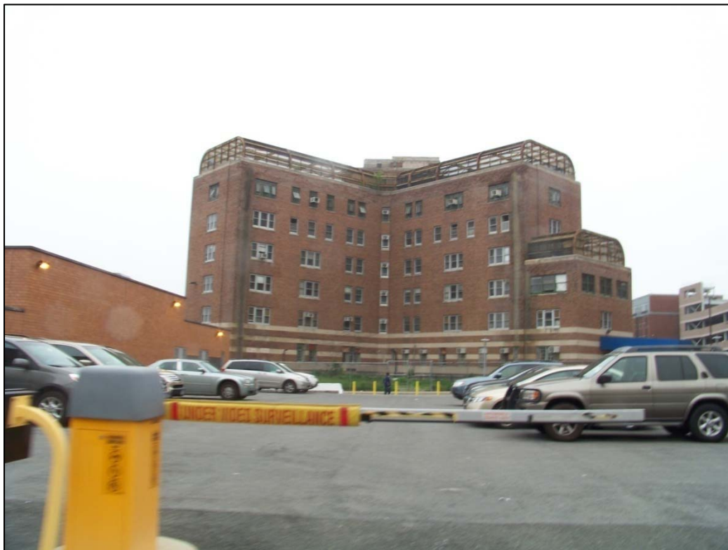
Photo 2: Building G (project site) from the West
