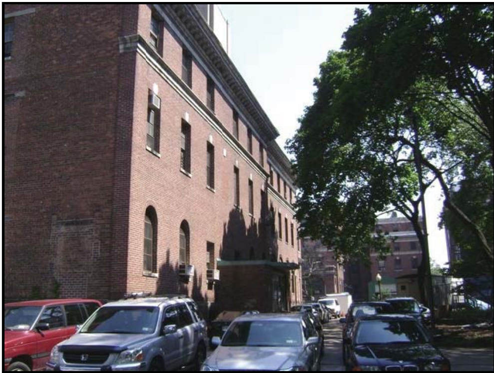
Photo 2: Rear (west façade) of Building J
