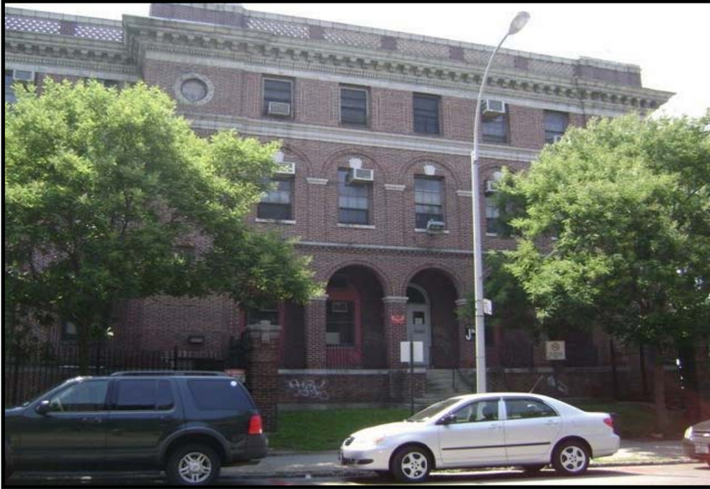
Photo 1: Building J from East
