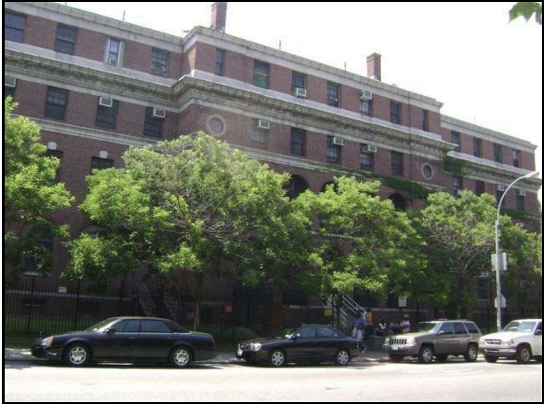
Photo 5: East façade of Building N
