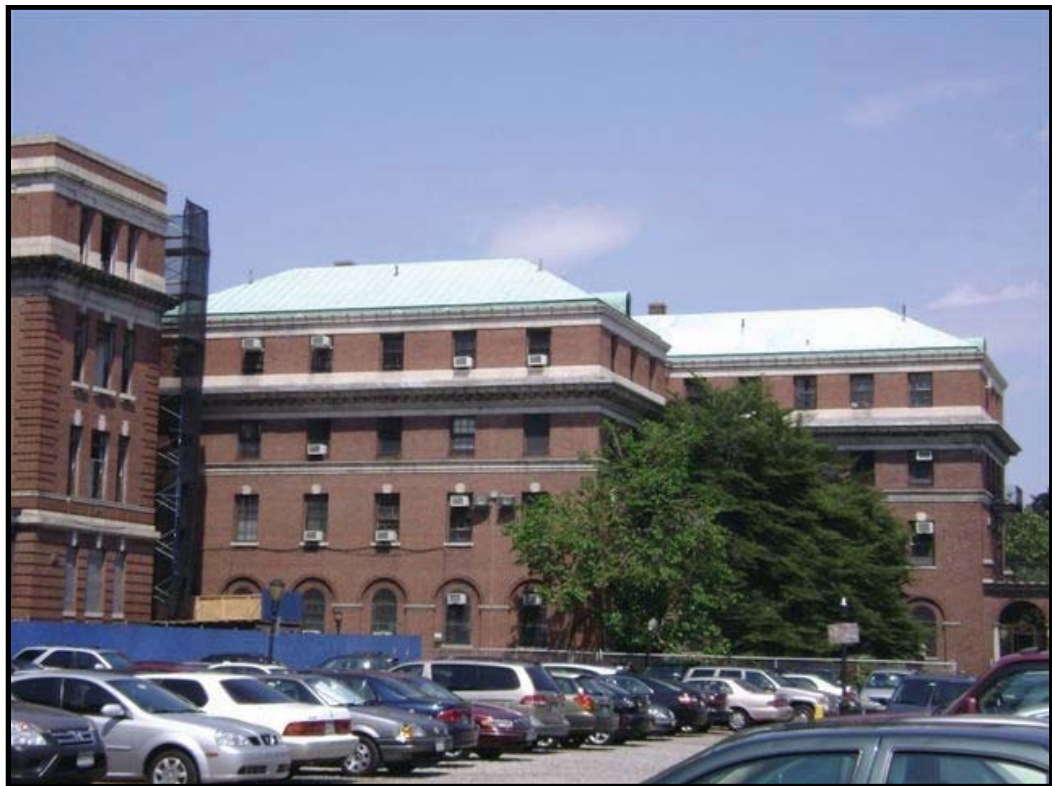
Photo 6: Rear (west) façade of Building N
