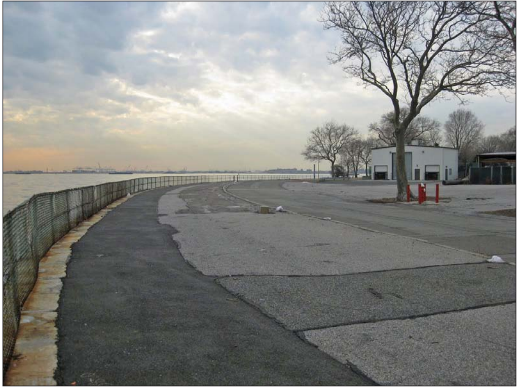
View west of southern tip of Island (South Island) 9
