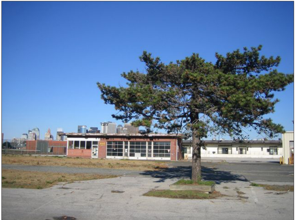
View northeast of motor pool building (South Island) 8
